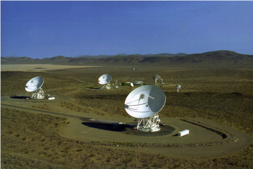
Figure 3: NASA’s Deep Space Network (DSN) dish array at Goldstone, California. During Artemis II’s trans-Earth coast, DSN stations provide the tracking data flight controllers use to determine Orion’s state vector and detect small trajectory deviations. Credit: NASA/JPL-Caltech.
